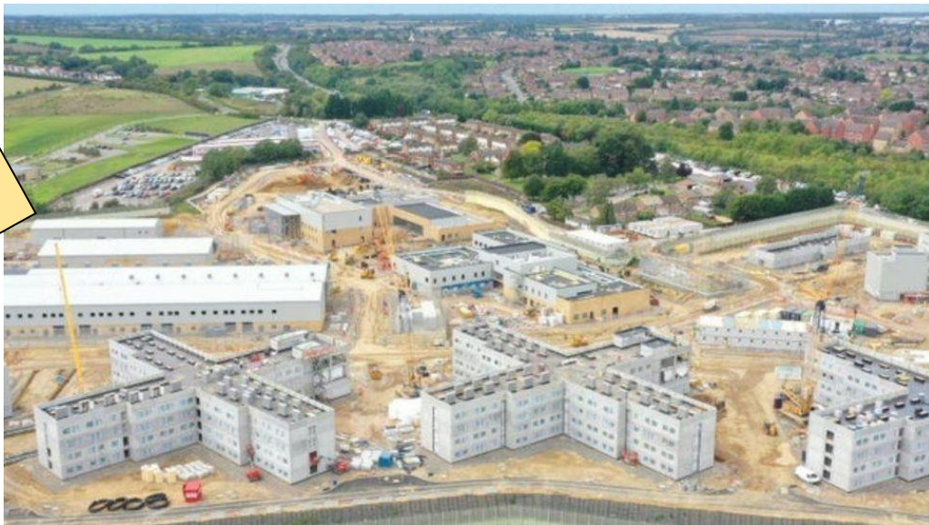
The new prison being built at Wellingborough
